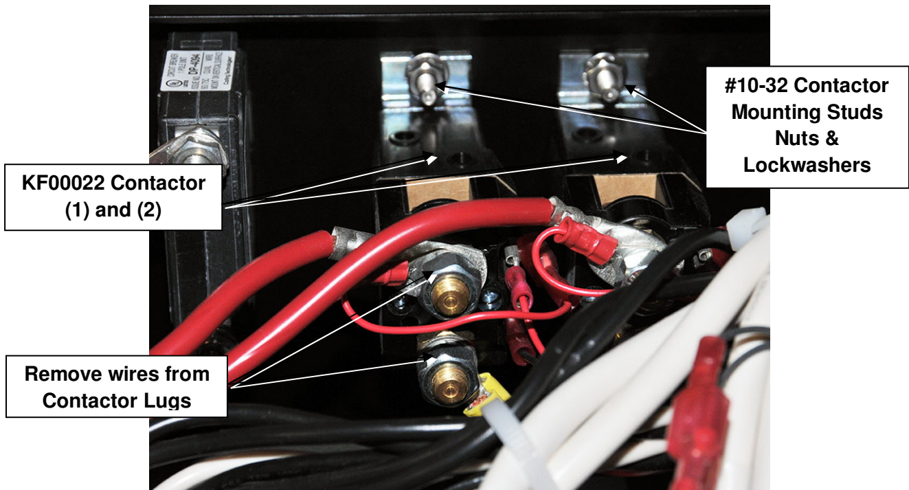
Figure 19: Replacing Contactors from Rear
