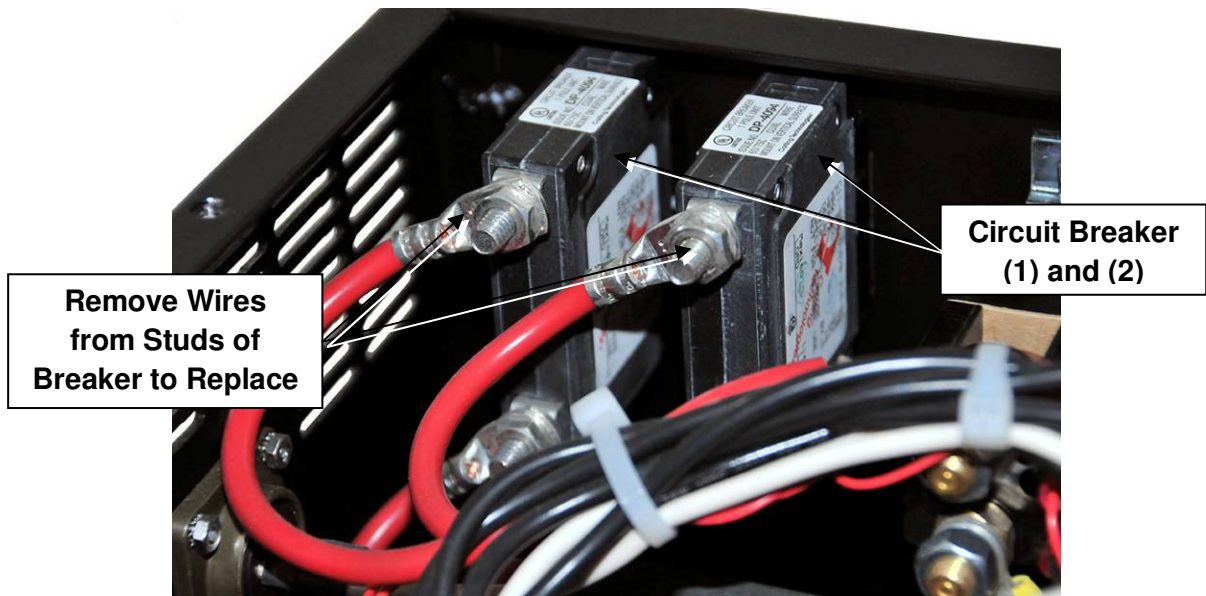
Figure 18: Removing Rear Wires of Circuit Breaker
